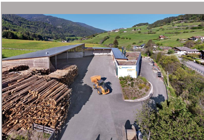
The biomass district heating plant. Source: Energy cooperative Villnöss
