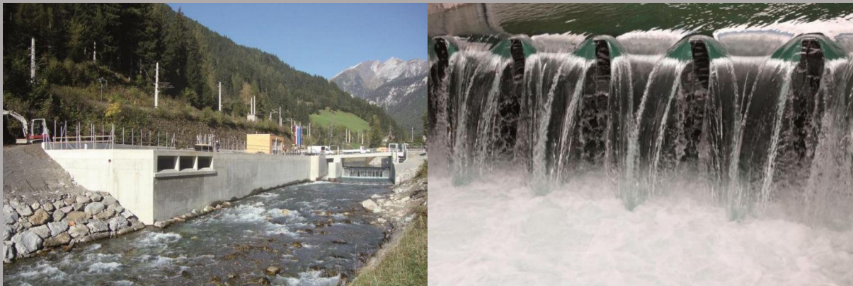
Pictures: Power plant (left) and fish ladder (right)
