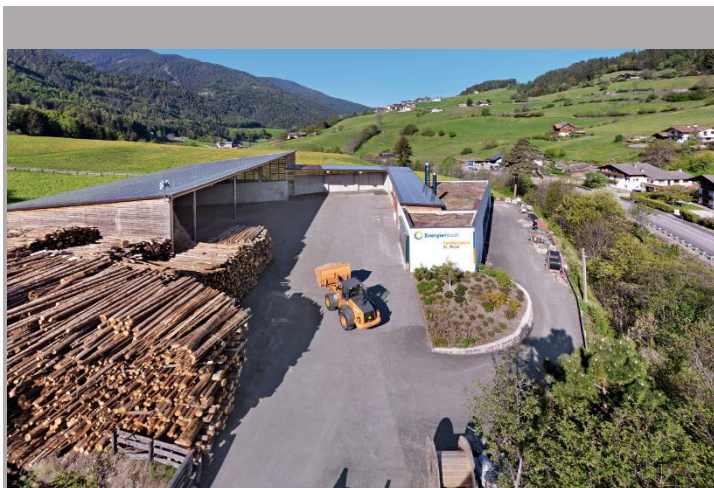
The biomass district heating plant. Source: Energy cooperative Villnöss
