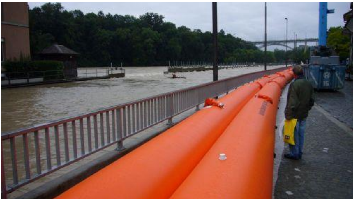
Figure 7: Beaver tubes as a mobile measure of intervention in the quarter of the “Matte” in the city of Berne © Professional fire brigade of the city of Berne, 2007
